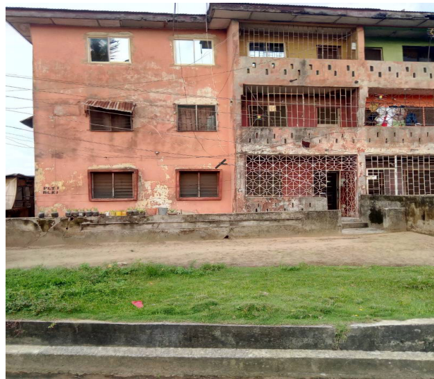
Plate 2: Poor building appearance at Ijaiye Housing Estate, Ojokoro, Lagos
