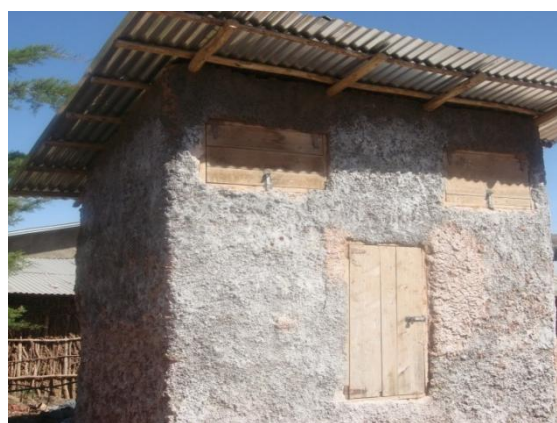
Figure 1: Potato tuber storage warehouse.
