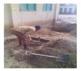
Plate I: Pits to access the foundation
