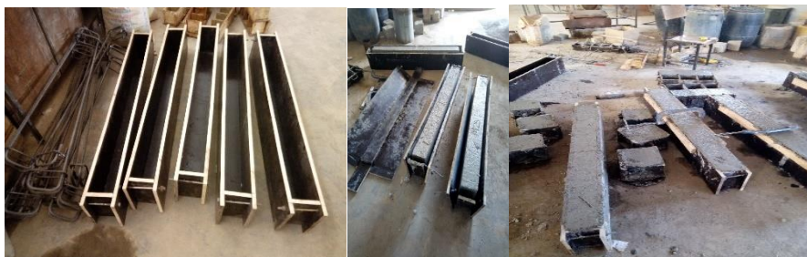
Figure 3: Wooden Formwork, Cast Beams and Cubes
