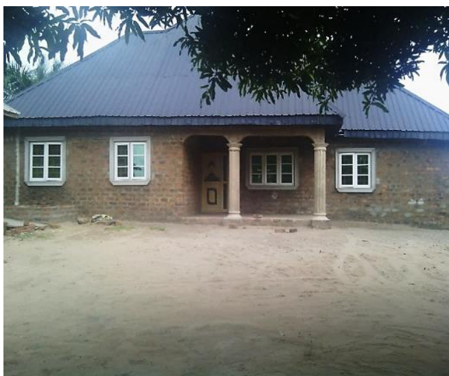
Figure 1: Three bedroom bungalows constructed with Makurdi local burnt bricks (a) without rendering; (b) with rendering
