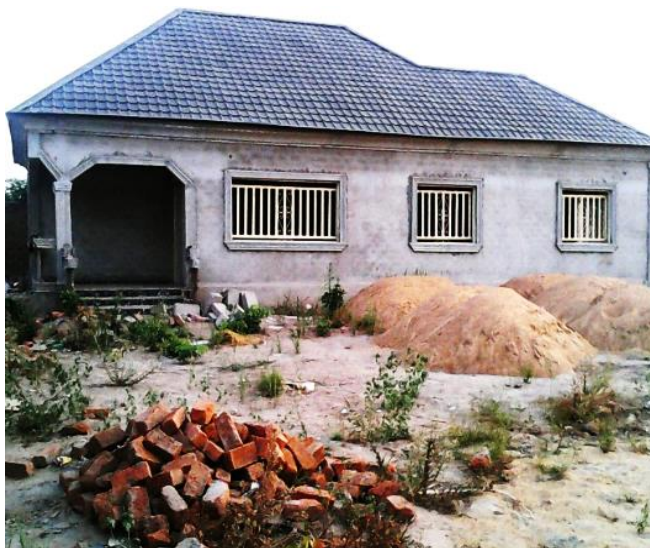
Figure 1: Three bedroom bungalows constructed with Makurdi local burnt bricks (a) without rendering; (b) with rendering
