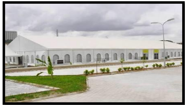
Plate VII; Temporary structure of Cunningham Marquee Event Centre, Abuja. (Source [18])
