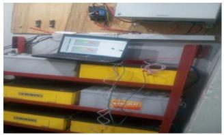
Fig. 4: Monitoring System Connected to PV Power Bank
