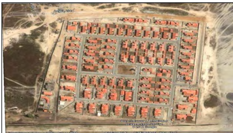
Fig 1.2 Satellite Image of Goshen Beach Estate (Google Earth, 2004)
