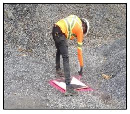
Fig. 5 Establishment of Ground Control Point
