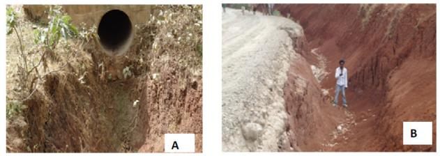
Figure 3: The gully associated with culvert (A) and the gully associated with roadside ditch (B) Characteristics of Gully Erosion
