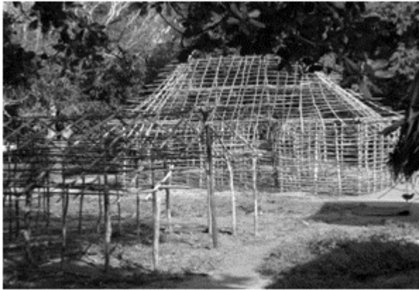
Figure 7: House construction using poles
