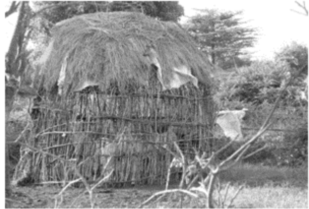
Figure 8: Kraal constructed using poles, grass and shrubs
