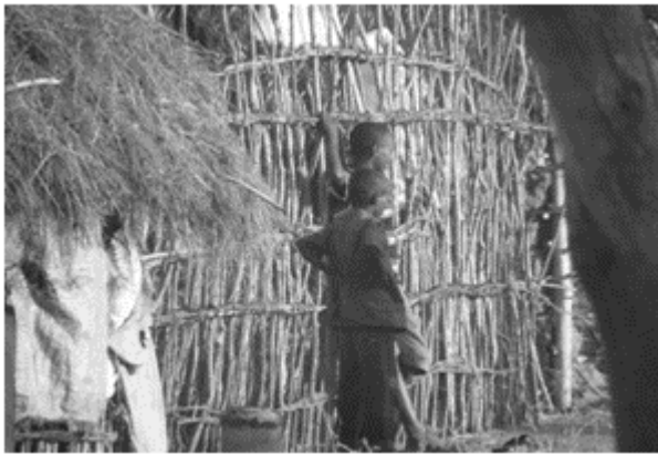
Figure 9: Fence demarcation using saplings and grass as roofing material
