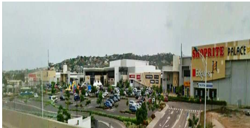
Fig. 3: View of the West Hills Mall from the N1 Highway
