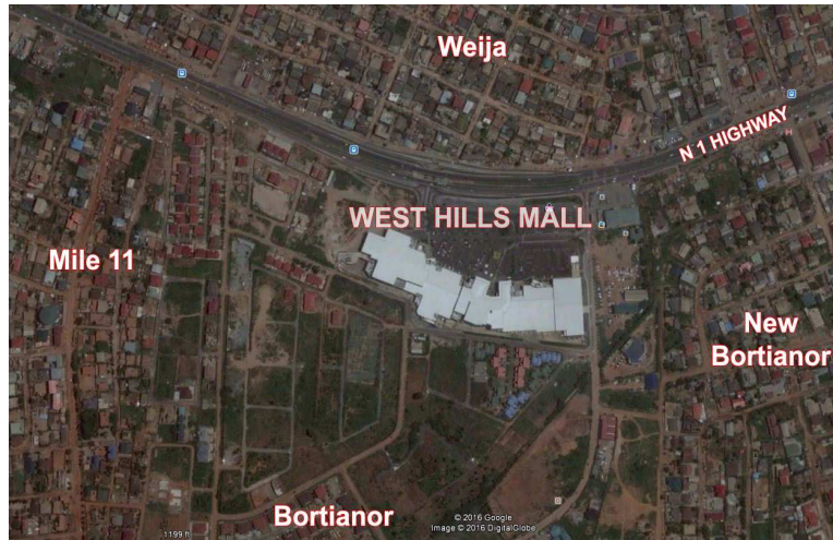
Fig. 2: Aerial view of West Hills Mall (Source: Google Maps, 2016)
