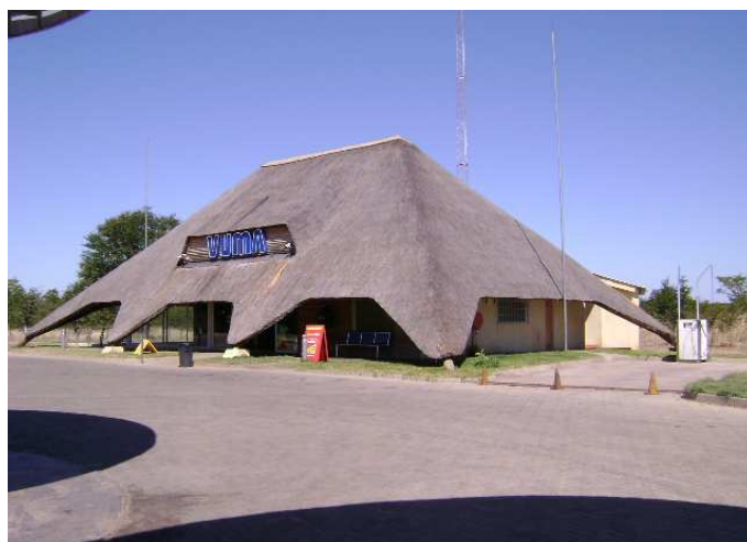
Fig. 3: A fuel filling station in Livingstone, Zambia roofed with thatch (Source: Authors')
