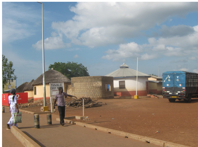
Fig. 2: Thatch roofs and mud walls of the Tamale Chief's Palace are gradually changing into metallic roofs and sandcrete walls (Source: Authors')
