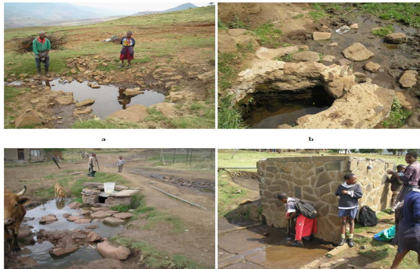
a = unprotected spring, b = open well, c = poorly protected spring and d = concrete covered protected spring
