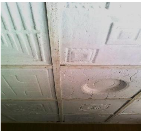
Plate 3: Fibre cement ceiling boards in application
