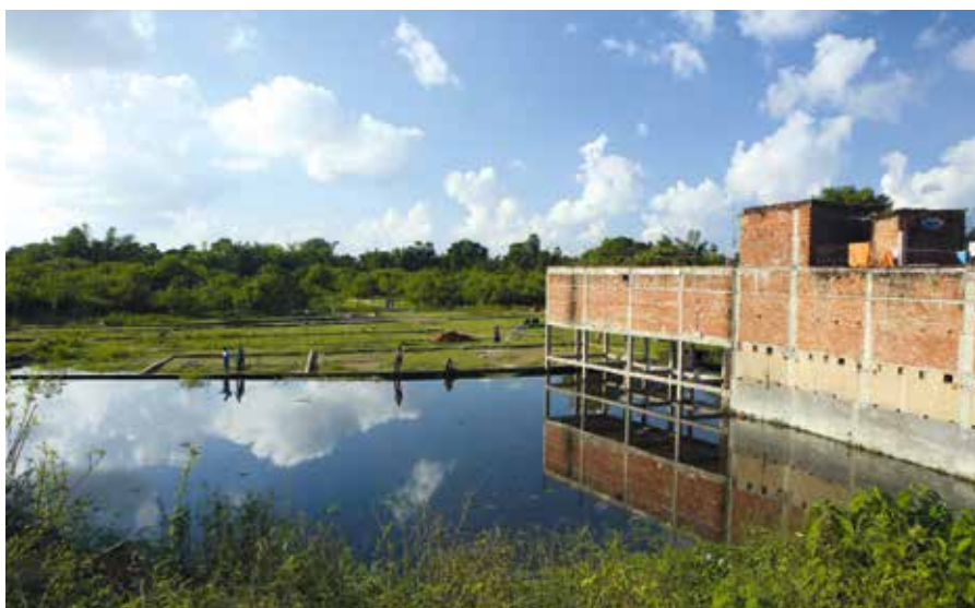
Construction in waterbody in peri-urban areas of Gorakhpur. Photo: GEAG
