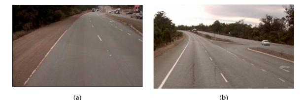
**Figure 1.** Examples of pavement markings in poor condition. (**a**) Edge line (left side) is worn down and even missing; (**b**) turning arrows and continuity line (right side) are blurred.
