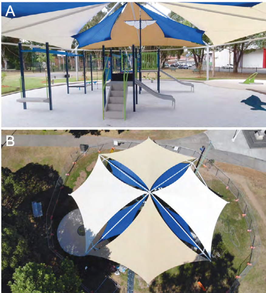
FIGURE 28: View of the shade sails from (A) below and (B) above the playground in Memorial Park. Differences in colour, position and venting gaps are clearly visible. Please refer to text for more details.
