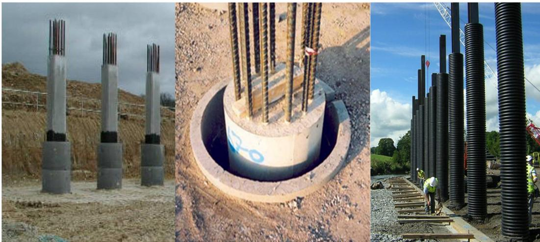
**Figure 6.** Sleeves around the piles.
