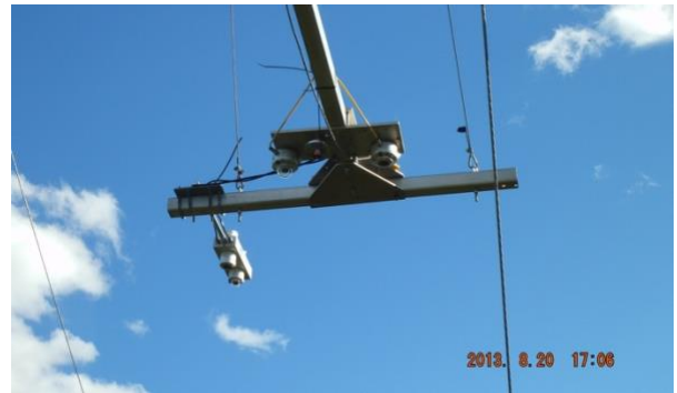
CNR1 (bottom view) along with downward looking pyranometer and pyrgeometer
