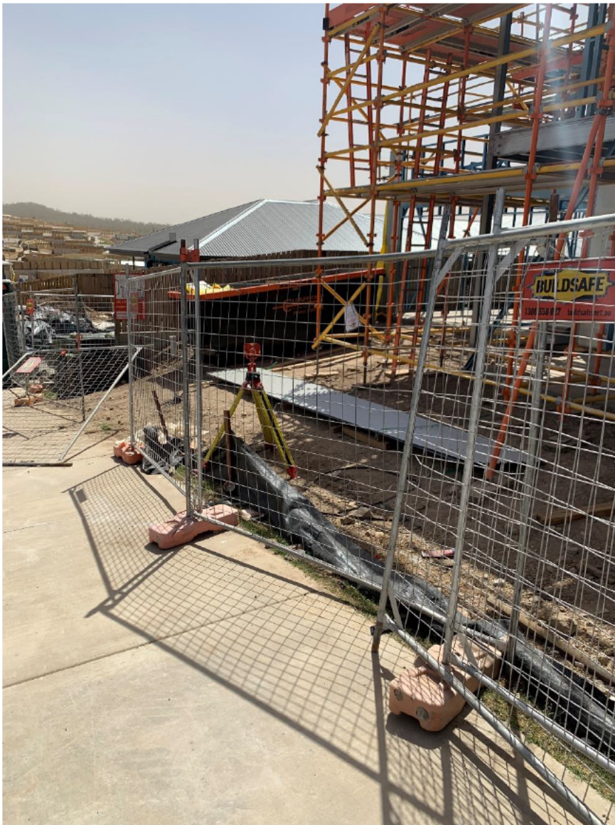
Figure 4.10, Experiment 10 – Temporary Construction Fencing
