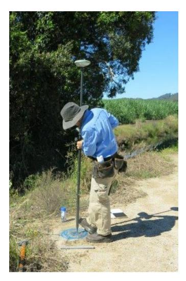
Figure 19: Placement and GNSS observation of control points
