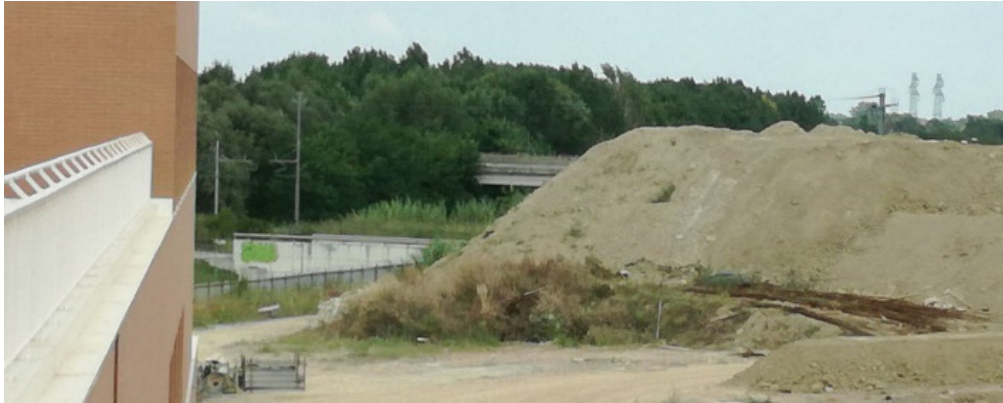
Fig. 7.3 The artificial hill created to protect the building from pollution coming from the railroad and the highway.
