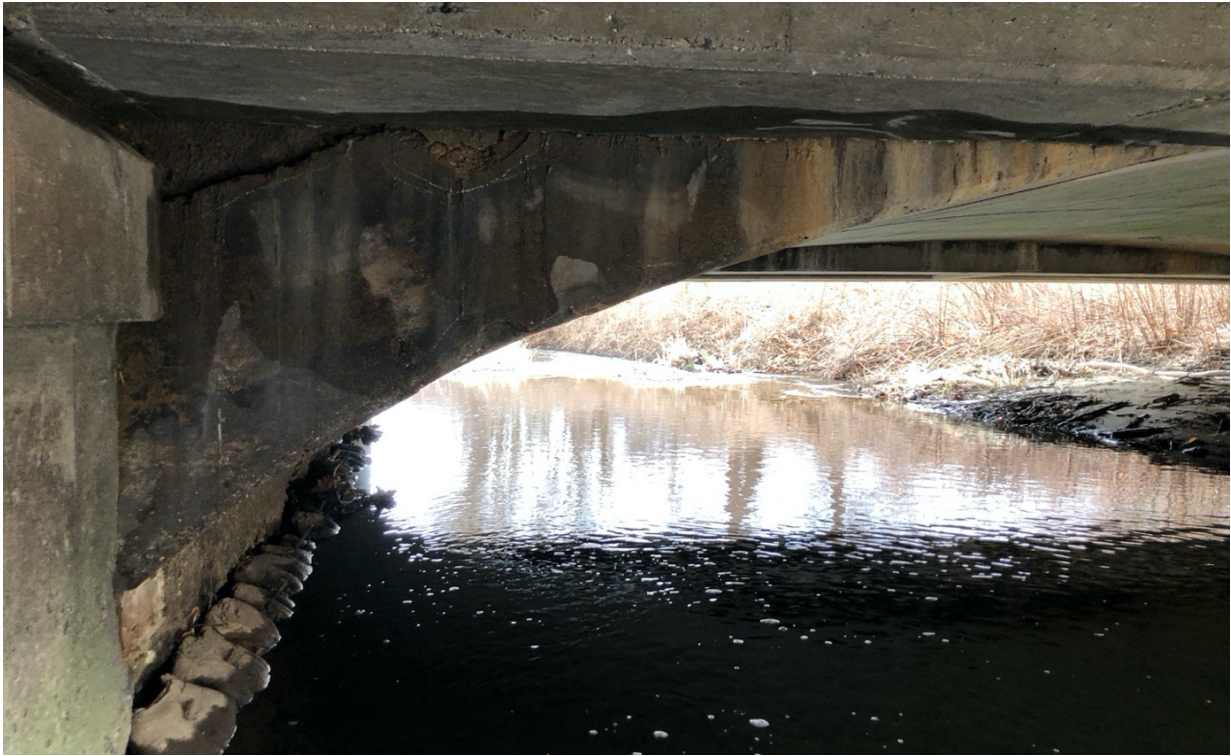
Figure 8.9: Northeastern haunch of the arch, January 2021.
