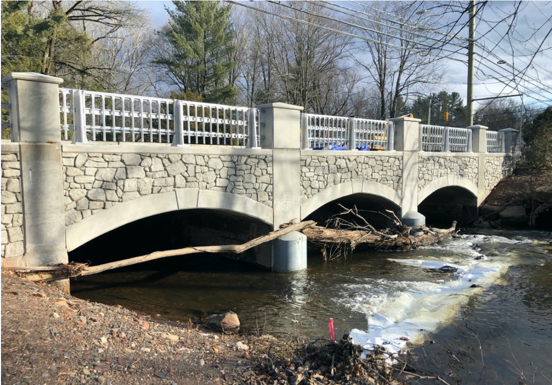
Figure 6.8: The west spandrel wall after reconstruction, January 2021.
