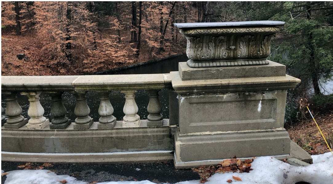
Figure 4.8: White Bridge Balustrade, January 2021.
