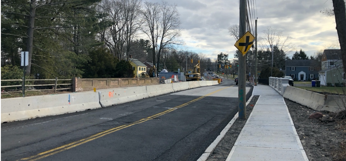
Figure 6.9: The roadway looking south with temporary Jersey barriers, January 2021.
