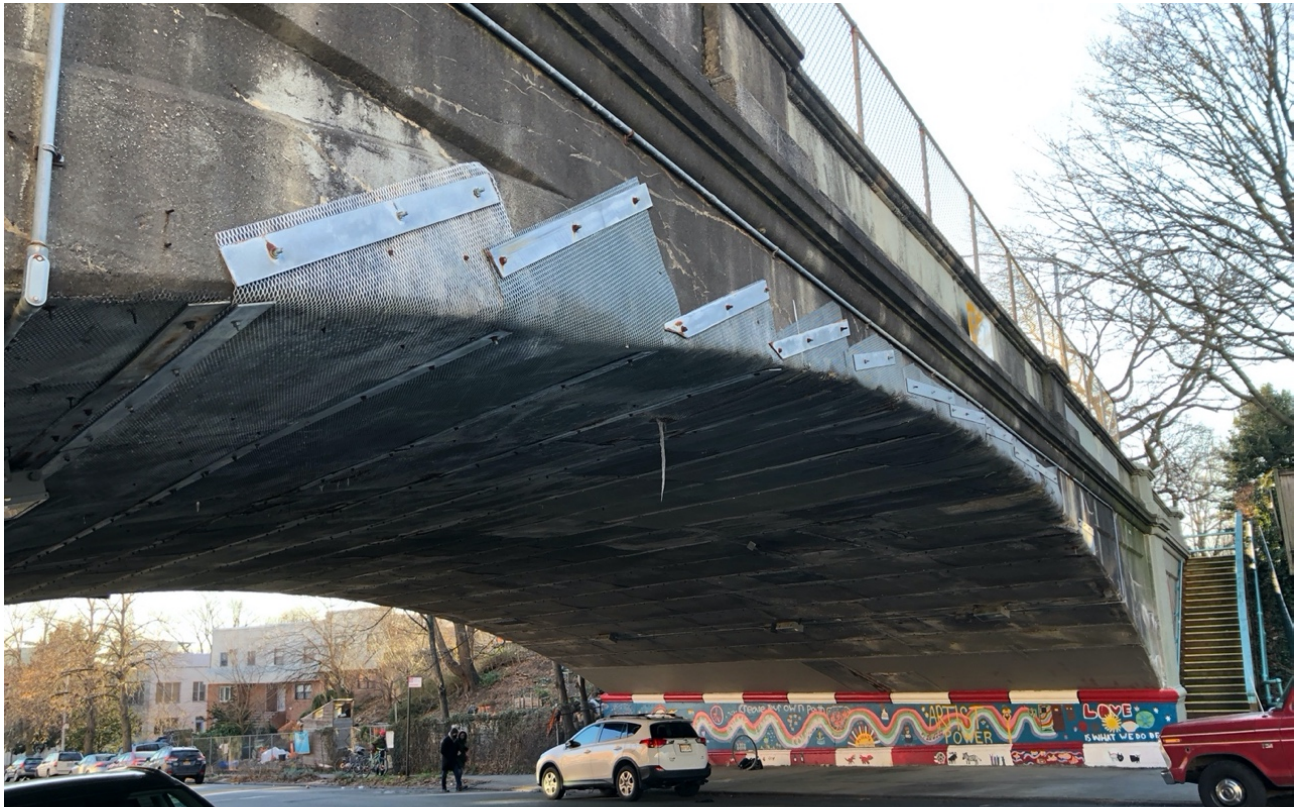
Figure 7.10: Steel netting covering the intrados, facing southwest, January 2021.
