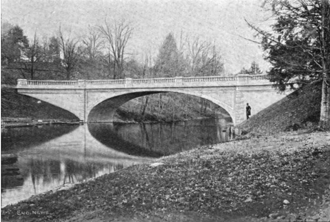
Figure 4.1: The White Bridge, Hyde Park, N.Y. (1897). Source: Engineering News , November 10, 1898, 290.
