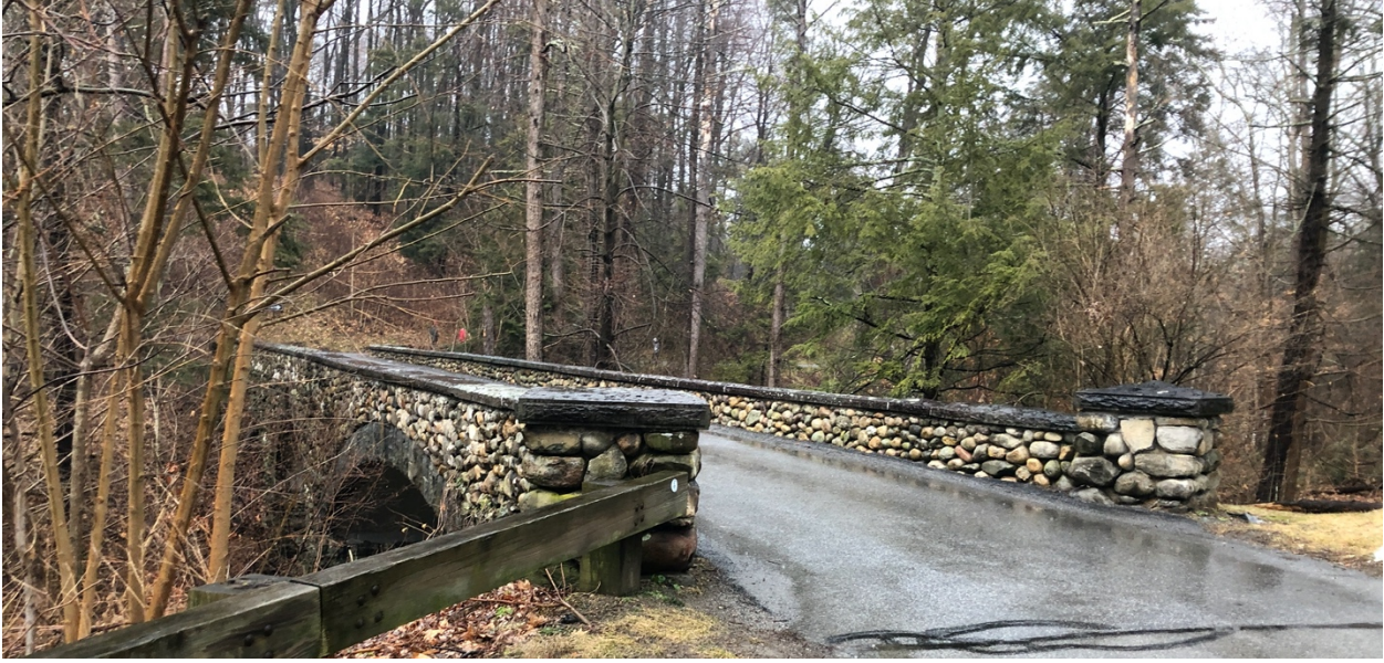
Figure 4.11: Coach House Drive over the Coach House Bridge, January 2021.
