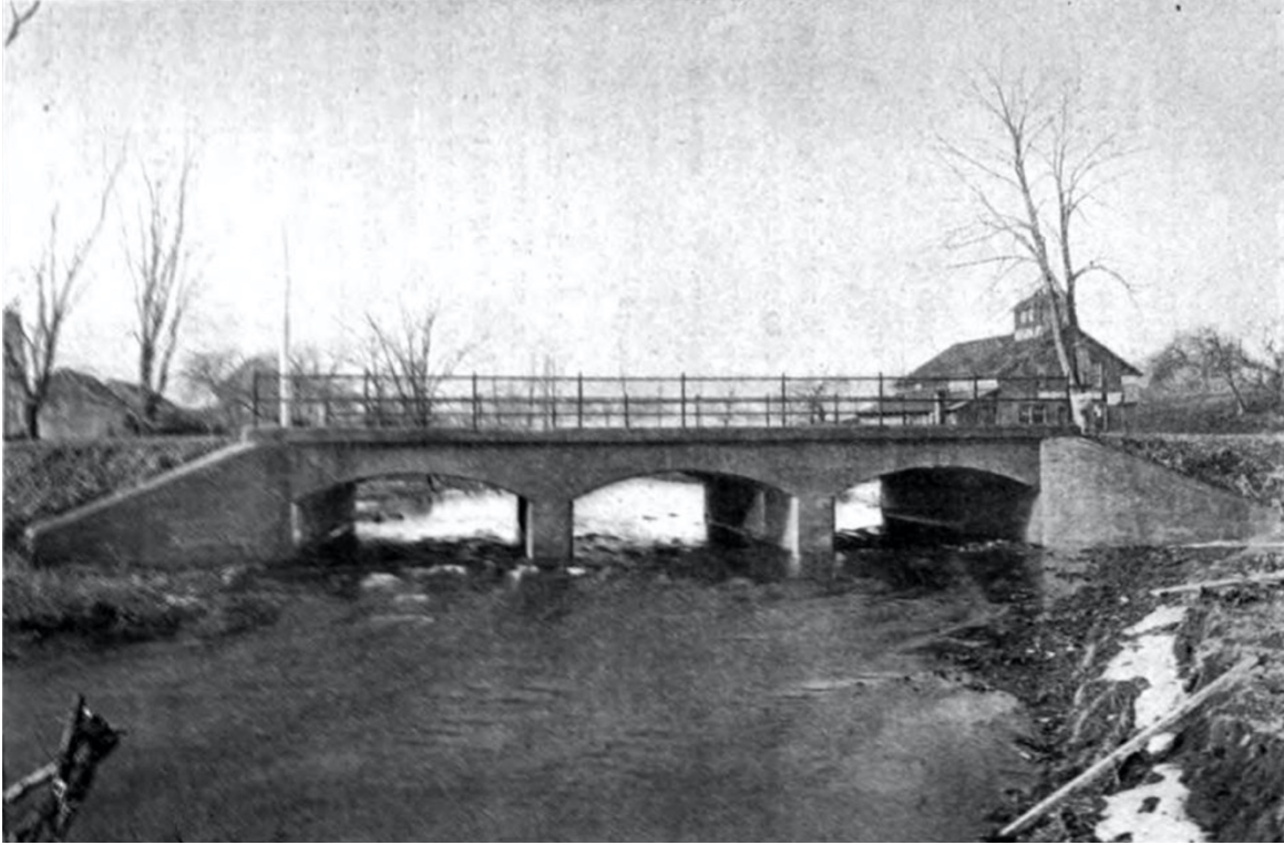
Figure 6.2: The North Main Street Bridge in 1901. Source: Town of West Hartford, we-ha.com
