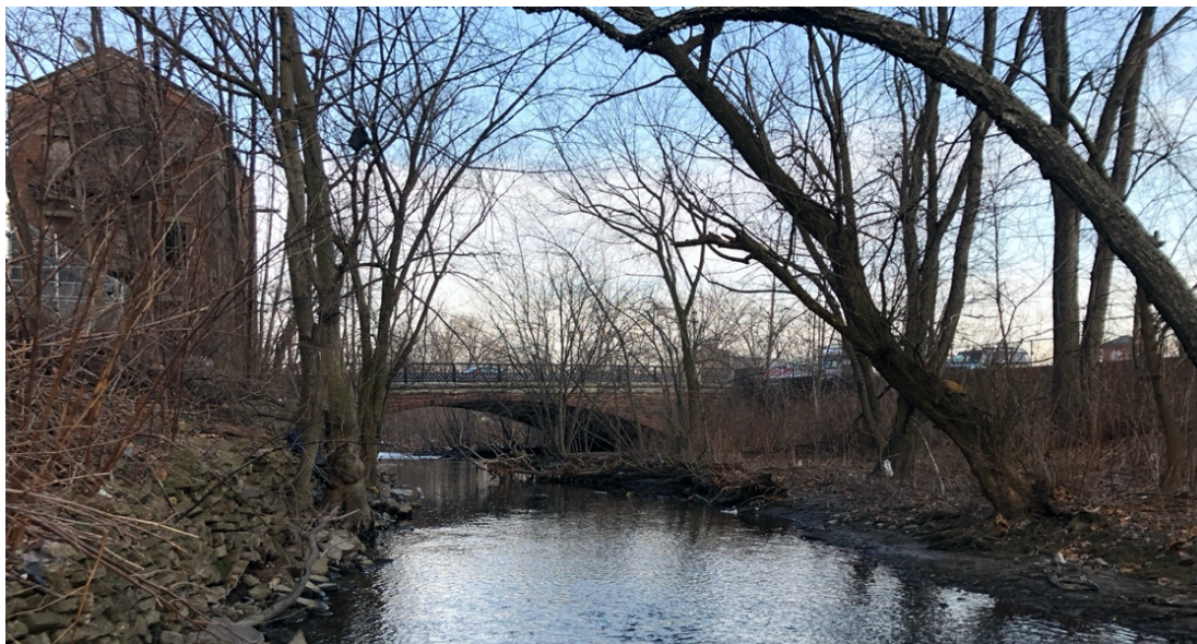
Figure 5.5: The northwest side of the West Broadway Bridge, January 2021.
