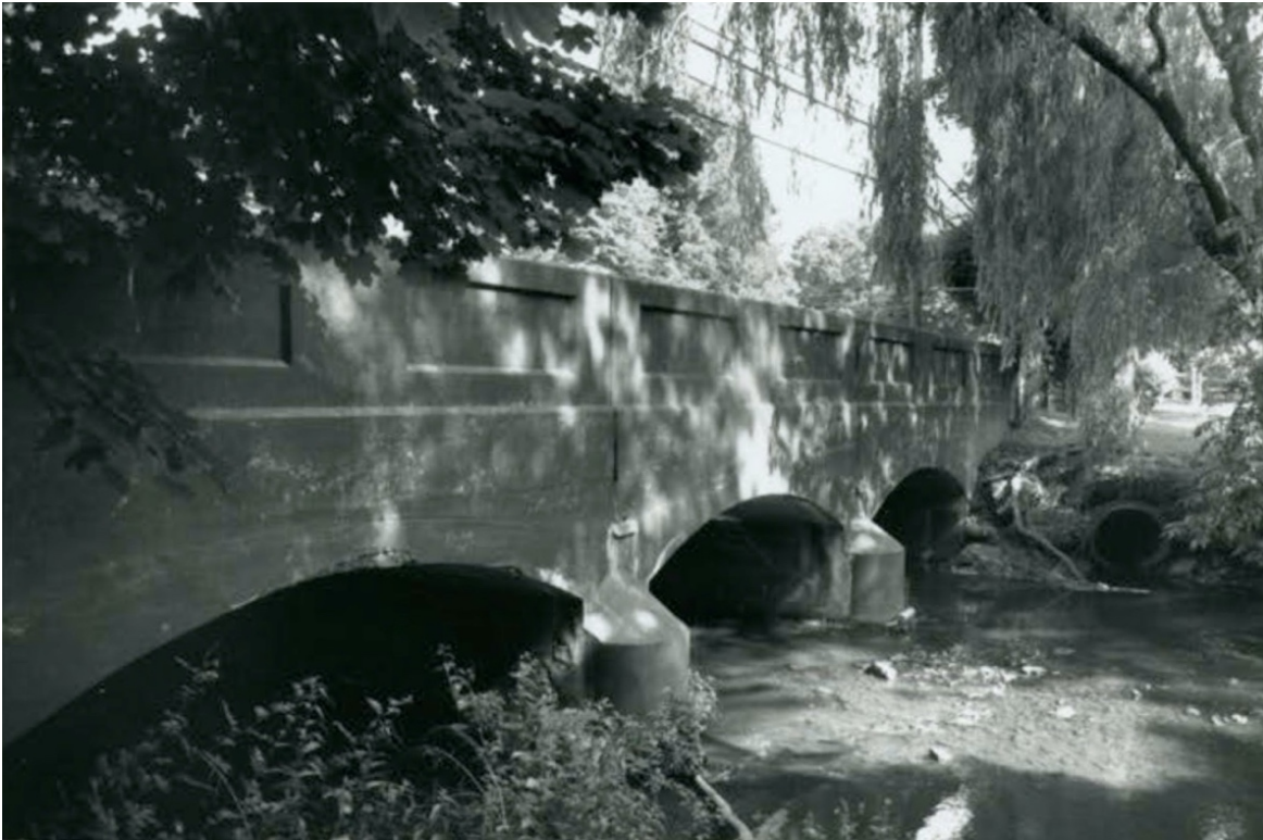
Figure 6.6: The western spandrel wall, photographed in 1990. Source: 1990 CT DOT Historic Bridge Inventory Report, Bridge 3651.
