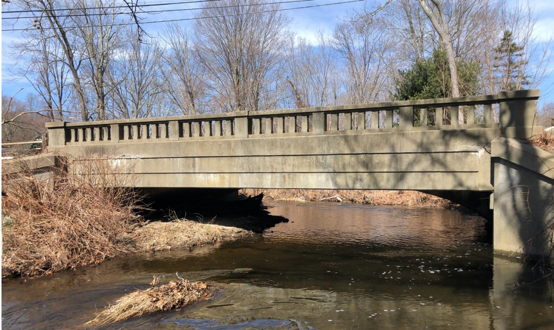
Figure 8.1: View of the South Façade of the bridge, March 2021.
