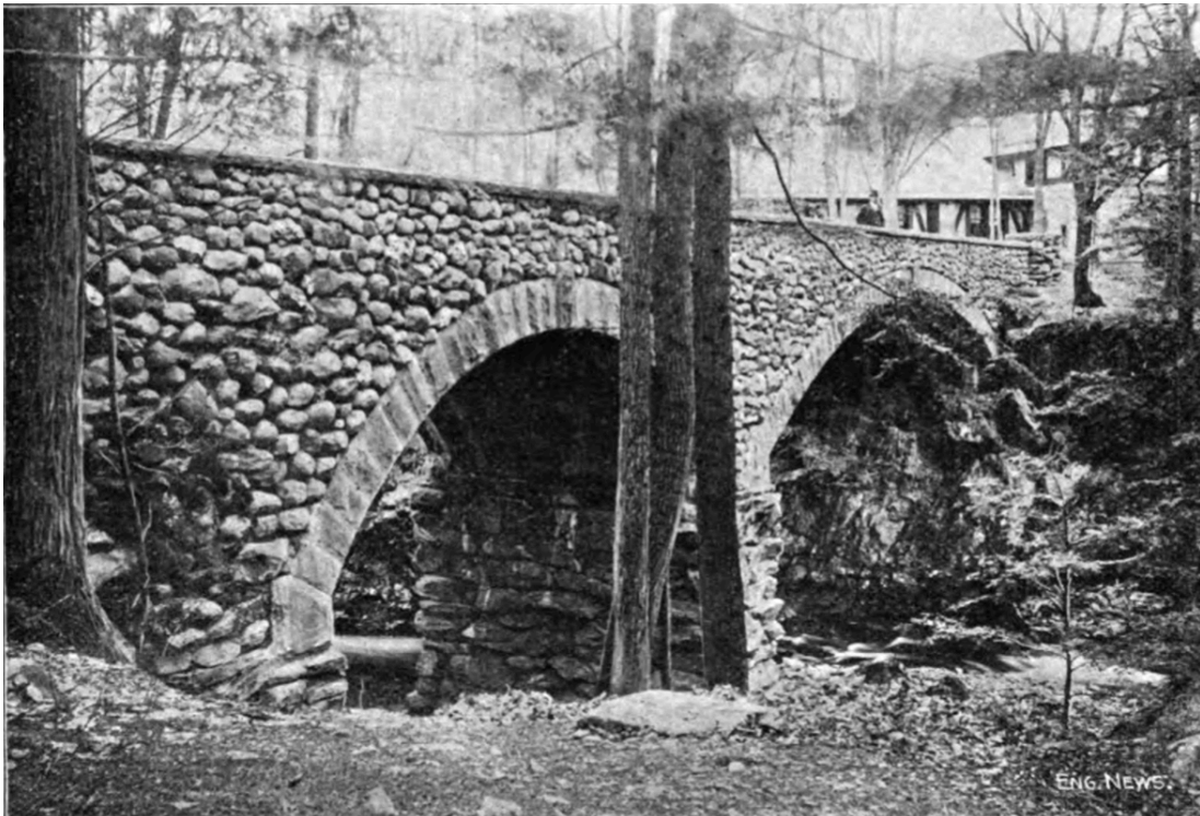
Figure 4.2: The Coach House Bridge, Hyde Park, N.Y. (1897). Source: Engineering News , November 10, 1898, 290.
