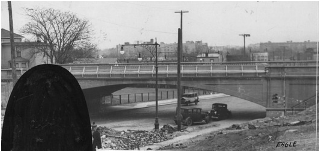
Figure 7.8: Photo of the north side of bridge, labeled 1932. Source: Brooklyn Public Library, Brooklyn Collection.
