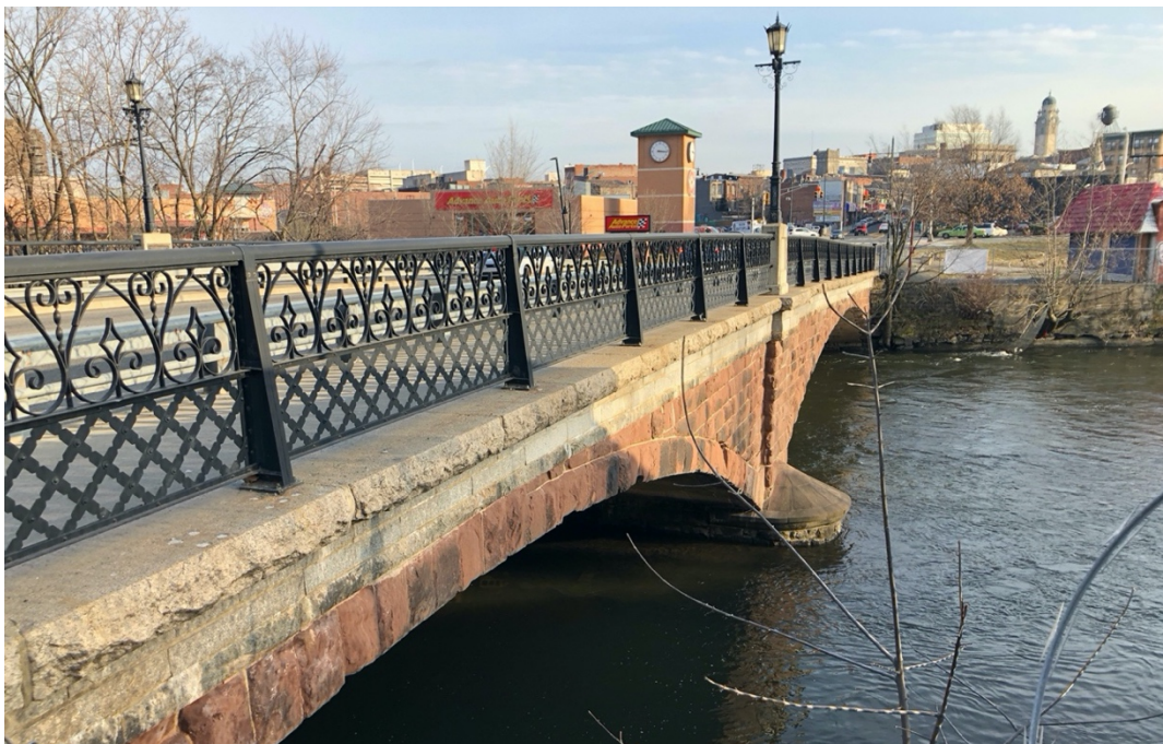
Figure 5.7: West Broadway Bridge, central and southern spans, January 2021.
