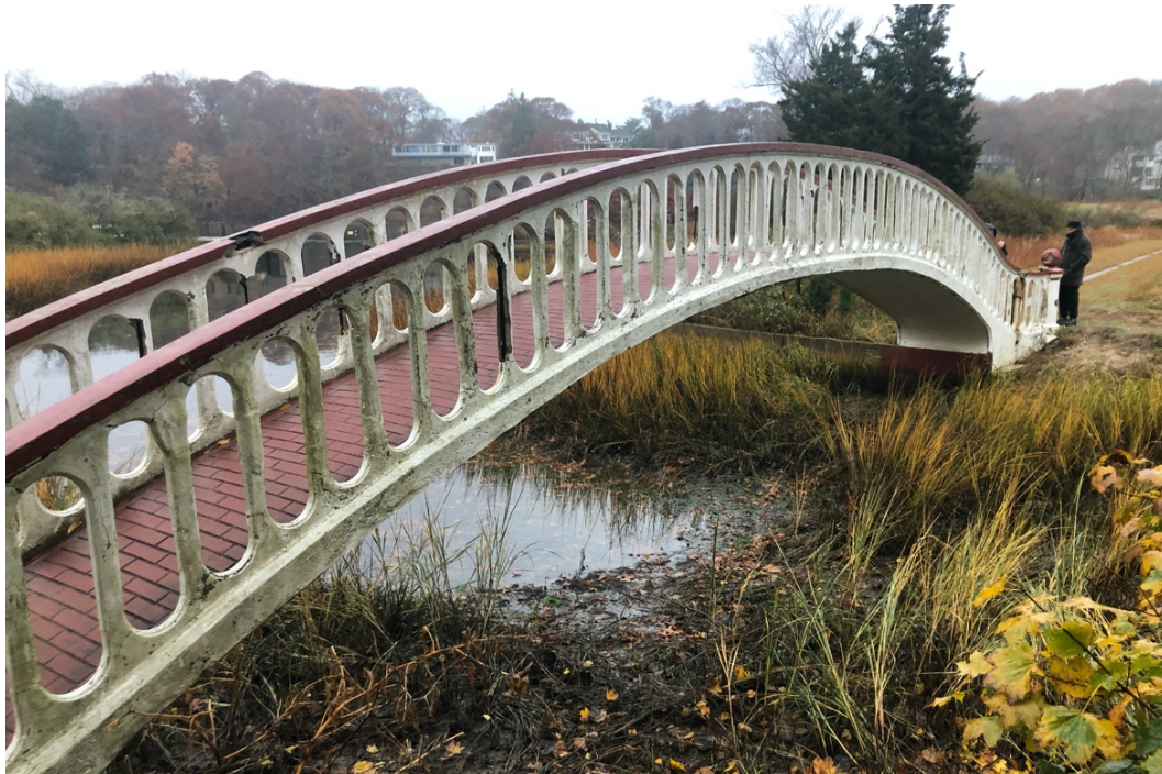
Figure 7: View of the bridge, November 2020.
