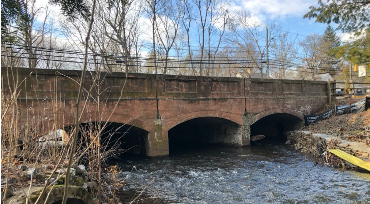
Figure 6.1: The eastern side of North Main Street Bridge, January 2021.
