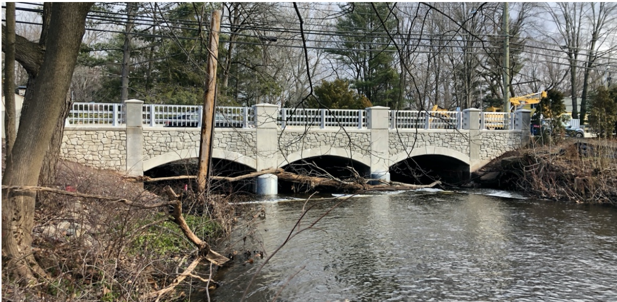
Figure 6.10: The west side of the bridge after reconstruction, January 2021.
