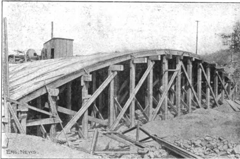
Figure 7.5: Wooden forms used for construction. Source: Engineering News , December 31, 1903, 588.
