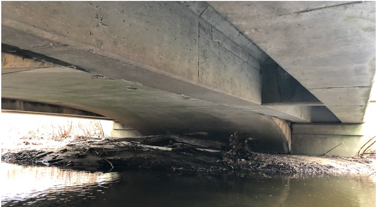
Figure 8.7: The underside of the bridge, facing west. January 2021.
