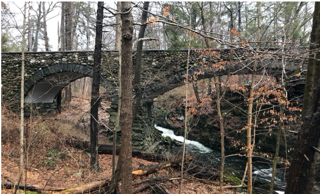
Figure 4.10: Coach House Bridge, January 2021.
