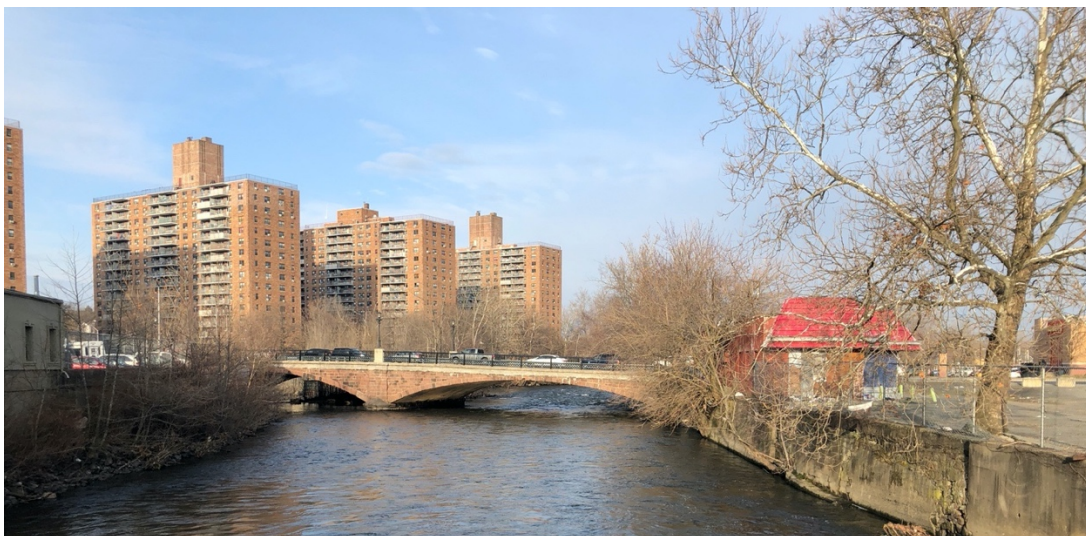
Figure 5.3: A portion of the southwest side of the West Broadway Bridge, January 2021.
