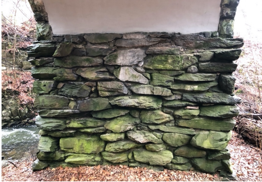
Figure 4.14: The Coach House Bridge Pier, January 2021.
