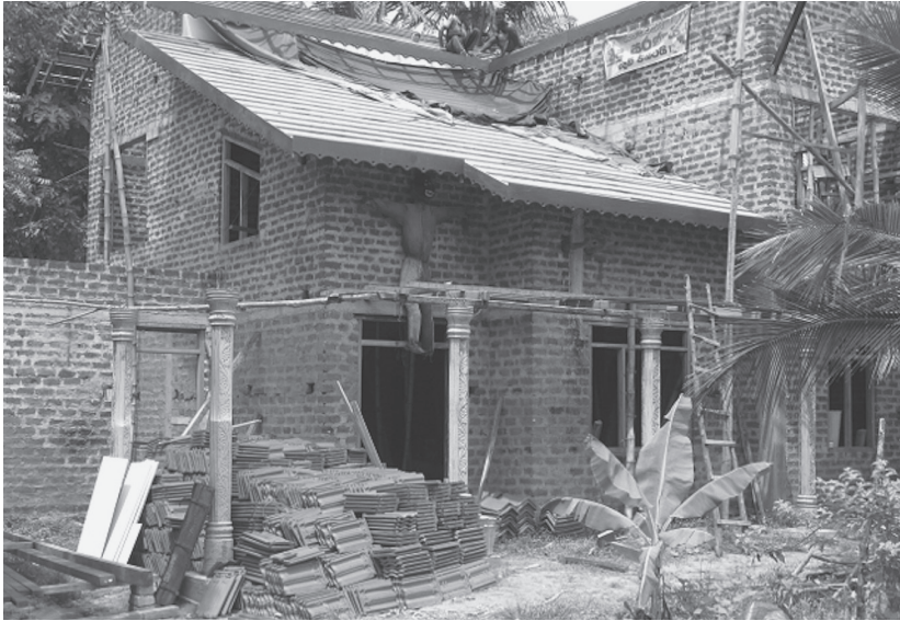
FIGURE 11.4. Walangama two-story house under construction in 2013. Adding a second story increases the number of hierarchical levels in the house's spatial syntax. (Photo: 2013, Deborah Winslow.)
