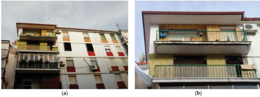
Figure 11. (a) Exterior façade of the dwelling under refurbishment; (b) Balcony façade detail.
