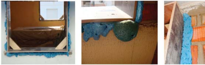
Figure 14. Special joints and high-durability flexible self-expanding polyurethane foam used.
