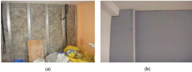
Figure 12. (a) Internal thermal insulation composite system; (b) Finished.
