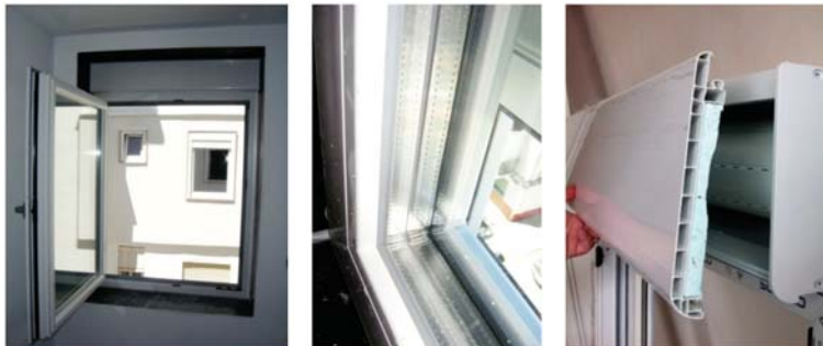
Figure 13. New façade windows.
