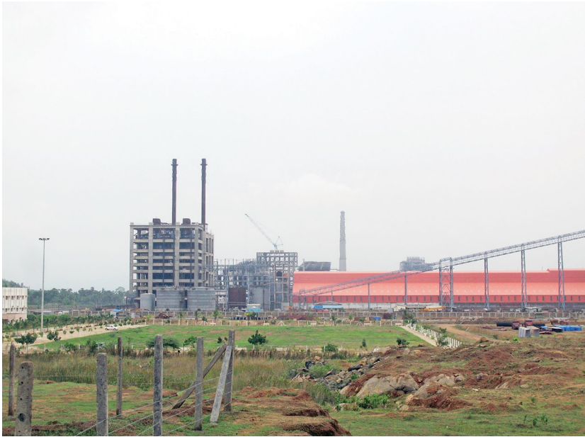
Figure 3.1 Construction of AnRak Aluminium's alumina refinery in Visakhapatnam District.
