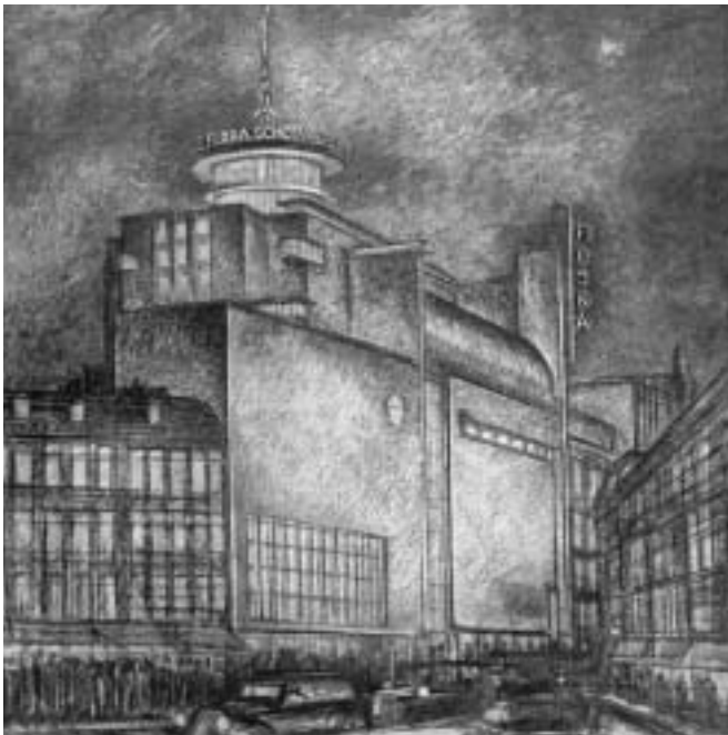
Fig. 68. Exterior of the Flora-Palace, designed by Jan Wils
