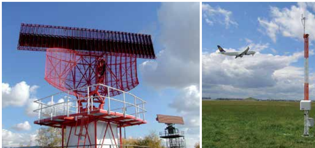
Fig. 1. Primary and secondary surveillance radar (picture source: author)
