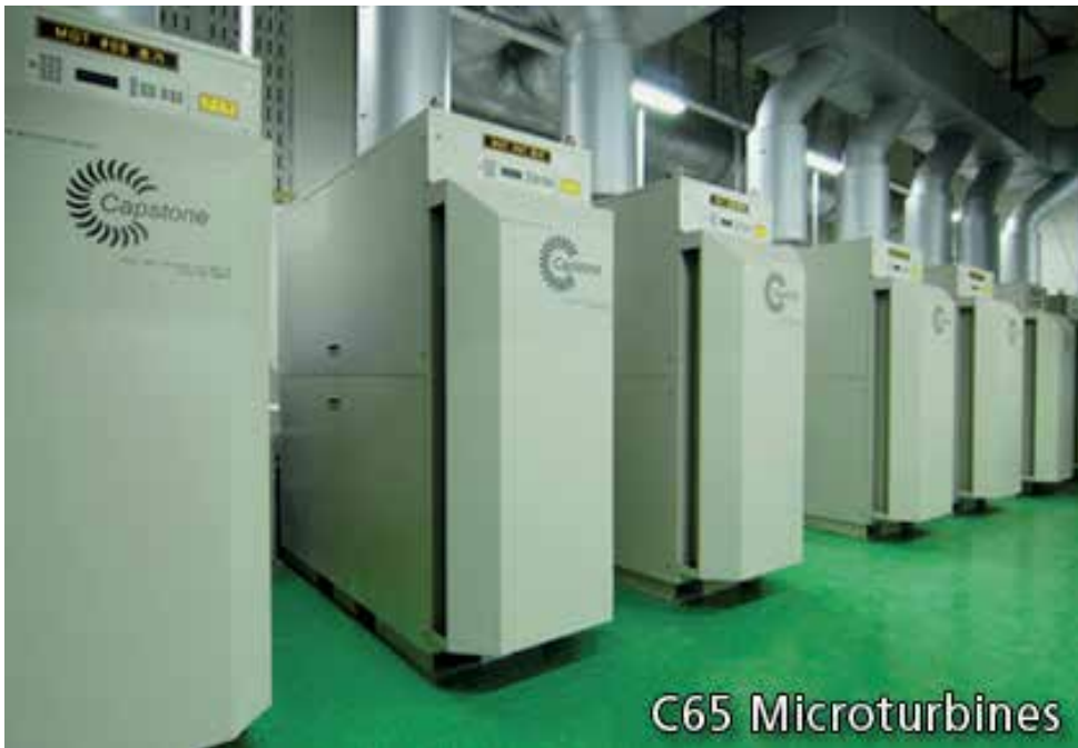
Figure 2. Capstone microturbine, model C65 (Capstone, 2012).
