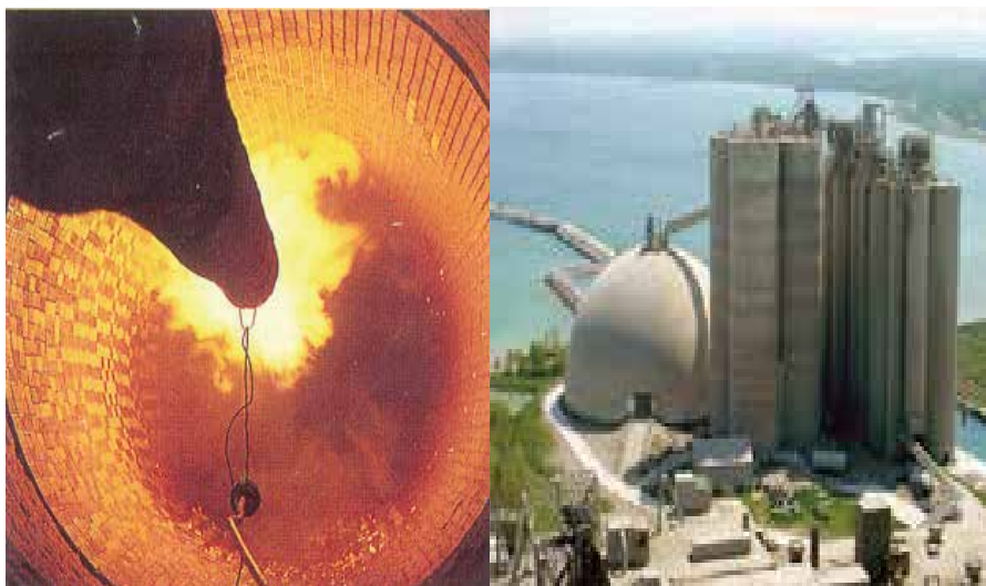
Fig. 6. Picture of inside (left) and outside (right) of a co-incineration unit in cement furnace used to burn dangerous industrial solid wastes (Puna, 2002).
