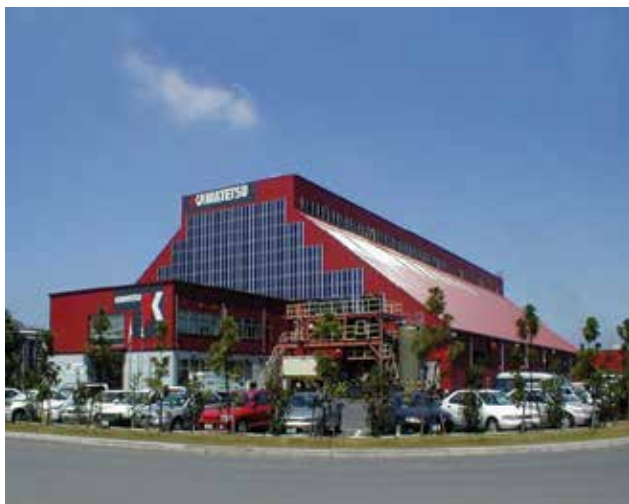
Photo 2. MSW gasification plant in Chiba (Japan)
