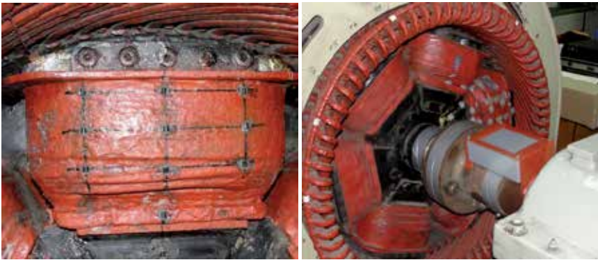
Fig. 23. Mounting of the temperature probes (left); measurement system in rotation (right)
