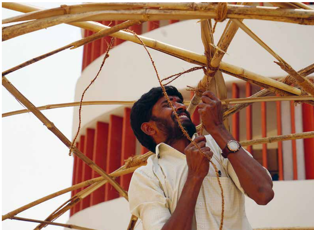
Constructing »Chhaya«. Photograph by L. Oppler, 2016
