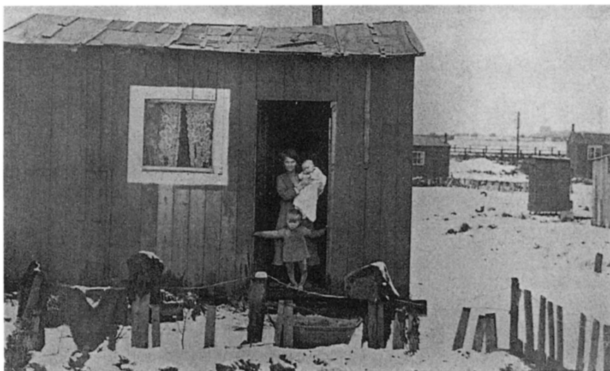
Figure 8.1b Accommodation for mine workers and families. The caption from this 1937 plate reads, 'Outside Newcastle: Whole families of miners live in these tiny and unsanitary dwellings, for which a rent of seven shillings is charged'. As with the previous photograph from Orwell's book, the photographer is unknown.
