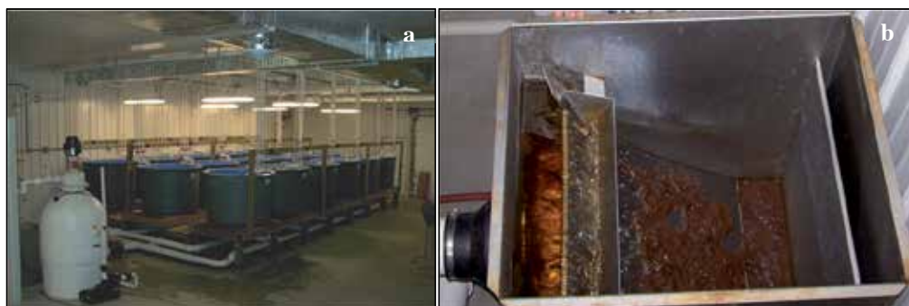
Figure 11. a. An indoor multi-tank recirculating aquaculture system (RAS); b. A parabolic screen filter in a RAS (Photo courtesy of Blank).
