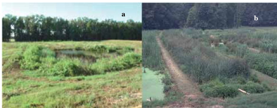
Figure 6. a. Settling basin. Picture courtesy of Auburn University; b. Constructed wetlands in Mississippi (Tucker 2009) (BMP No. 6 2002).
