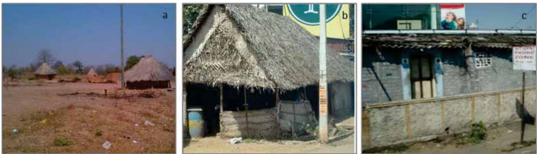
Figure 10. An estimated 90% of sub-Saharan buildings and housing are not lightning-safe, such as (a) farming settlement with thatch and sheet metal roofs on mud brick walls in Zambia, (b,c) combination shops and homes in India (©M.A. Cooper).
