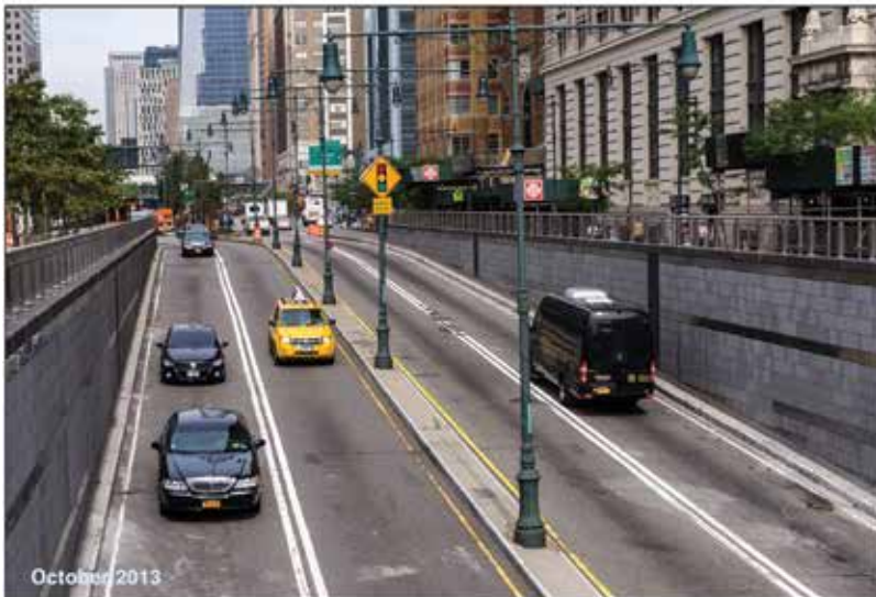
Battery Park Underpass - New York City, New York
