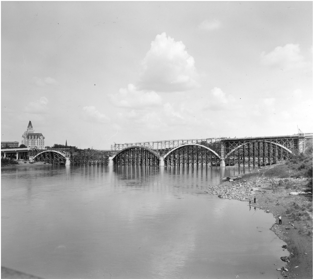
Figure 7. The arch work for the Broadway Bridge, 1932. When the photograph was taken, the bridge's official opening was just over two months away. City of Saskatoon Archives, 1104-003-050.
