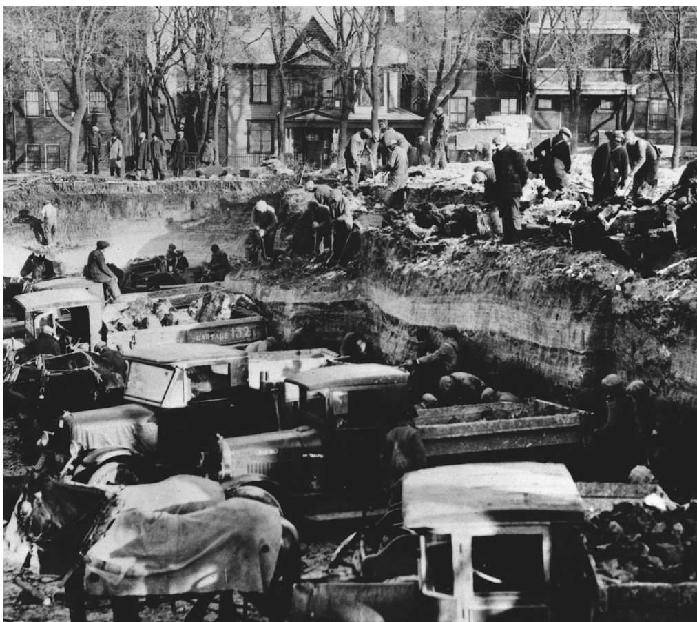
Figure 8. Relief workers in Winnipeg, 1931. Here, workers prepare the foundations of the site that will house the Civic Auditorium. The engineers who organized the project insisted on using as little construction machinery as possible. Relying on hand labour instead of machine labour meant that more men could find work on the project. Provincial Archives of Manitoba, Winnipeg – Buildings – Municipal – Civic Auditorium, Collection item 10, N9182.
