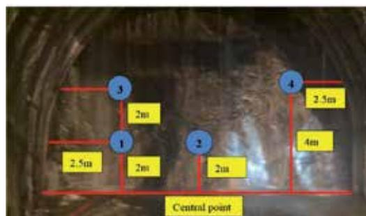
**Figure 5.** Position of the lead drilling hole.
