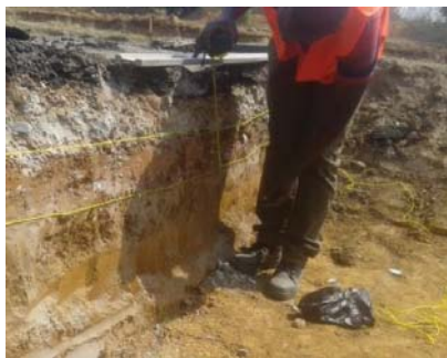
Figure 7. Trench measurements of Pit 3 (Kitwe-Ndola).
