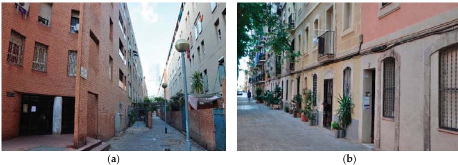
Figure 10. La Barceloneta: (a) social housing in MTM, and (b) small houses.
