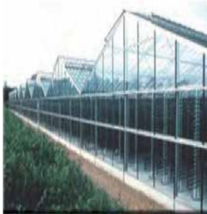
Figure 14. Glass tube photobioreactor (700 m 3 ) producing Chlorella biomass (Klötze, Germany)
