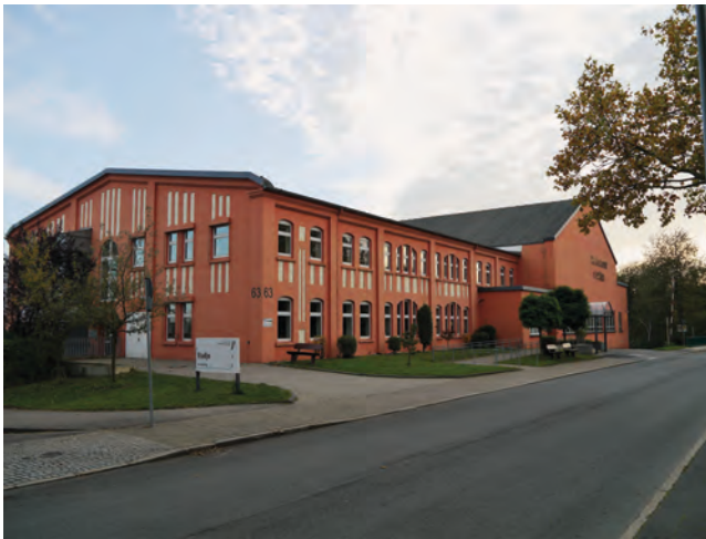
Figure 4.5 Former administration building and payroll office of coal mine Dannenbaum, now housing community centres and educational facilities.
