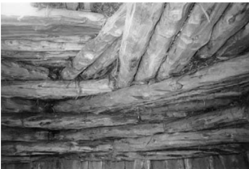
Fig. 5. Corbeled roof on female hogan interior. Photo by the author.
