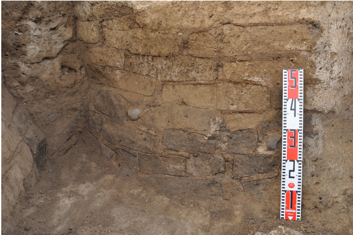
Fig. 3.29 Wall of Building 511 of Level 5 showing the use of mud-bricks with different colors. Yellowish-brown mud-bricks were laid above dark grey ones. Looking southeast.
