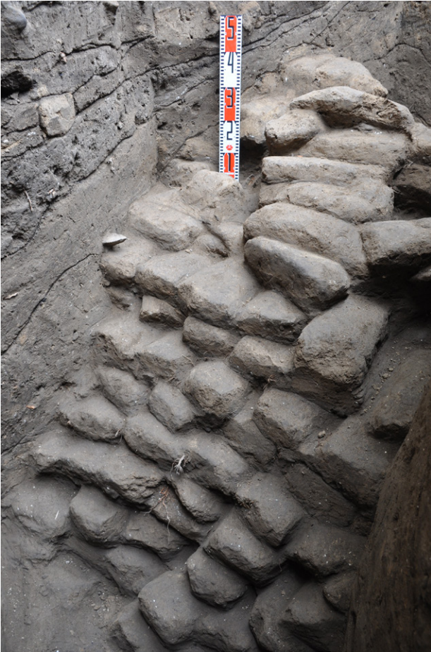
Fig. 4.51 Side view of the structure of Level 13 in the sounding pit of Square 4B, seen from the northwest.
