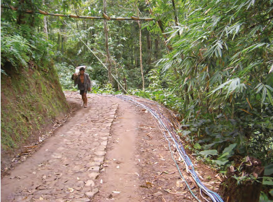
FIGURE 14 Clean water used to be transported by gutters made of lengthwise cut bamboo. This is gradually replaced by a system of PVC pipes lying on the ground. Path near Kaduketug 1, 11 December 2013
