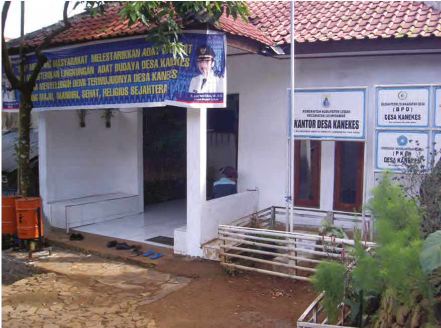
FIGURE 10 Office of the Kanékés secretariat in Cibolégér, about 100m from the residential house of the secular village head in Kanékés. 21 July 2016
