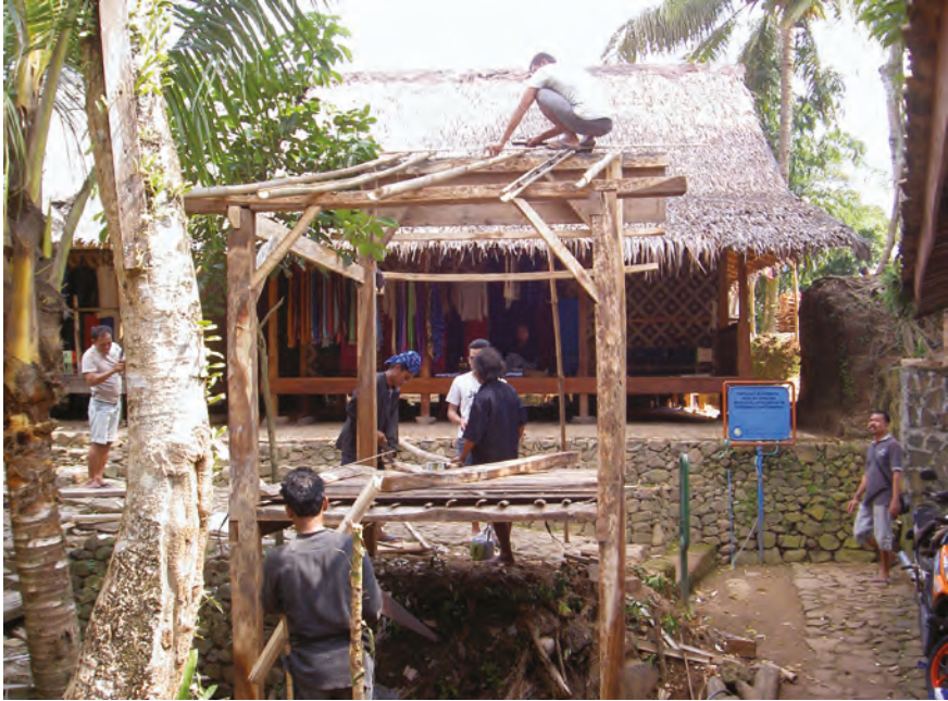
FIGURE 58 Baduy men building a new entrance post at Kaduketug 1, Kanékés, when entering from Cibolégér on the right. On the blue sign on the right visitors are asked to keep the environment clean from garbage. Kaduketug 1, 6 July 2016
