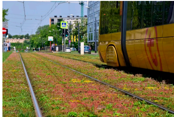
Figure 12. Warsaw: Grochowska Street, Praga district. The vegetation cover of tracks, mainly of Sempervivum L. and Sedum L. species—a very ornamental green carpet with extensive maintenance. Photo shared with permission: Warsaw Trams Llc., 2020 [65].
