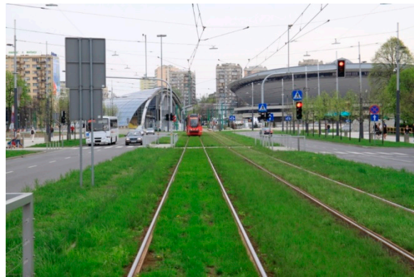
Figure 4. Poland, Katowice, W. Grassy tram lane along Kofranty Avenue. Photo: B. Fortuna-Antoszkiewicz, IV 2016.
