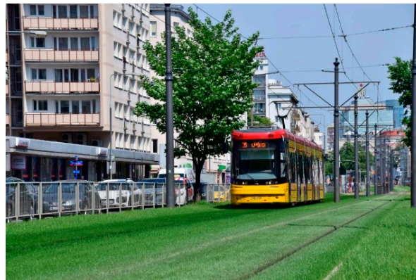
Figure 15. Warsaw: Puławska Street, Mokotów district. Smooth, grassy track cover gives a representative appearance to the main streets of the city. Photo shared with permission: Tramwaje Warszawskie Llc., 2020 [65].
