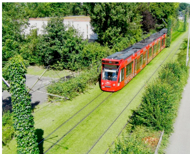
Figure 24. The tram train traveling in the “green corridor” consisting of grassy tracks, bordering trees, shrubs, and climbers attached to electric poles. Freiburg im Breisgau (Germany) has implemented numerous green tracks since 1980 [74].
