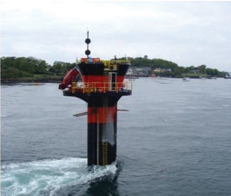
FIGURE 13.7 The world's first commercial scale and grid-connected tidal stream generator—SeaGen—in Strangford Lough. (Adapted from “Tidal power,” Wikipedia, the free encyclopedia, 2013.)
