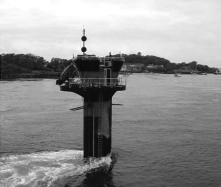
FIGURE 13.7 (See color insert.) The world's first commercial scale and grid-connected tidal stream generator—SeaGen—in Strangford Lough. (Adapted from “Tidal power,” Wikipedia, the free encyclopedia, 2013.)
