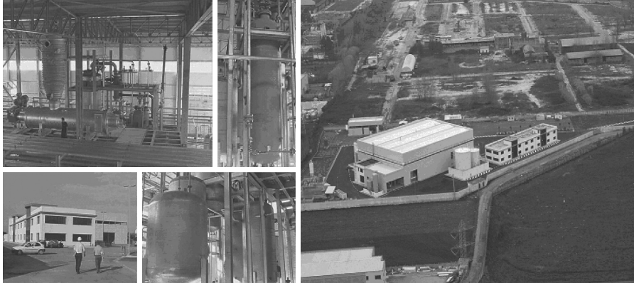
FIGURE 7.8 Commercial plant in Caserta, Italy. Recovery vessels (top left); outside of building (bottom left); mixing tank (top middle); second reactor (bottom middle); aerial view (right). (From “Fitzpatrick, S., Renewable chemicals and biofuels for sustainable bioplastics council of Maine ,” Paper presented by Biofine Technology, LLC, 2012. With permission; Hayes, D., Ross, J., Hayes, M., and Fitzpatrick, S., “The Biofine process: Production of levulinic acid, furfural and formic acid from lignocellulosic feedstocks,” in Biorefinery (8b) Industrial Processes and Products: Status Quo and Future Directions . Wiley, New York, 2008. With permission.)
