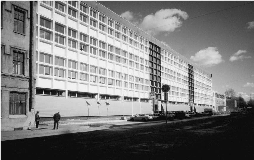
Figure 7.7 Sampsonievski hypermarket – post-transformational type of industrial buildings recycling
