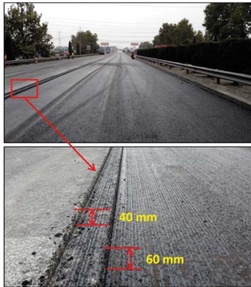
Figure 4. Treatment of underlayer surface with emulsified bitumen to ensure good bonding with the middle layer.
