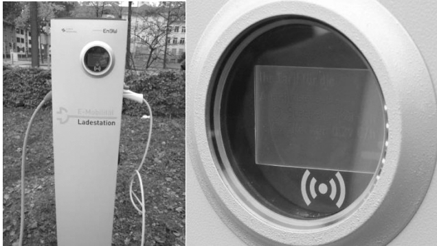
Figure 24: A public EVSE with two recharger cables (left), and the display enlarged with socket information (right).
